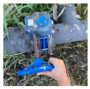
Ensure line is depressurized before working on the system. Complete regular maintenance and inspections.
