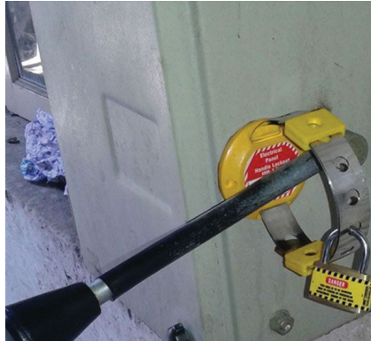
Electrical bar held in the off position
