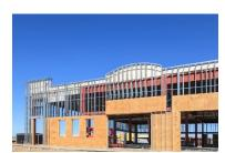
Class 5403: Exterior metal studs are light-weight and non-structural. Their primary purpose is to attach exterior shell or siding. 12-25 gauge steel.
